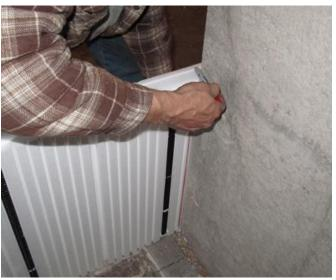
Mark and cut the panels about ¼" less than actual measurement needed so panels are not tight to the inside or outside corners, leaving a ¼" gap reduces the push out stress on the panels.
