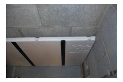
When you cut an InSoFast panel to fit into a corner the cut panel continuesturns or wraps around the corner.
