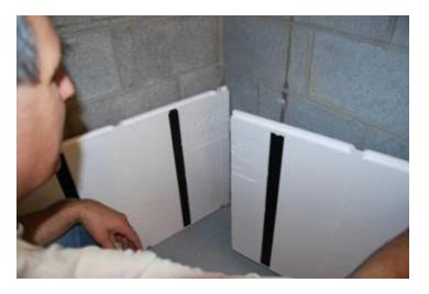
Mark and cut the panels about ¼" less than actual measurement needed so panels are not tight to the inside or outside corners, leaving a ¼" gap reduces the push out stress on the panels.
