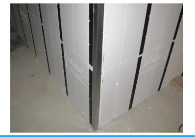
Apply a bead of adhesive directly on to the metal utility corner angle.
